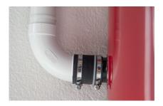
The suction port is on the bottom left of the central vacuum cleaner. Push the rubber sleeve and the other two hose clamps above the port.
