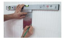
1. Align the wall bracket on the wall at the optimal height (approx. 1.60 m) and mark the drill holes on the wall.
