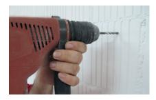
2. Using a 6 mm masonry drill, drill the five holes deep enough that the pins can be sunk fully into the wall.
